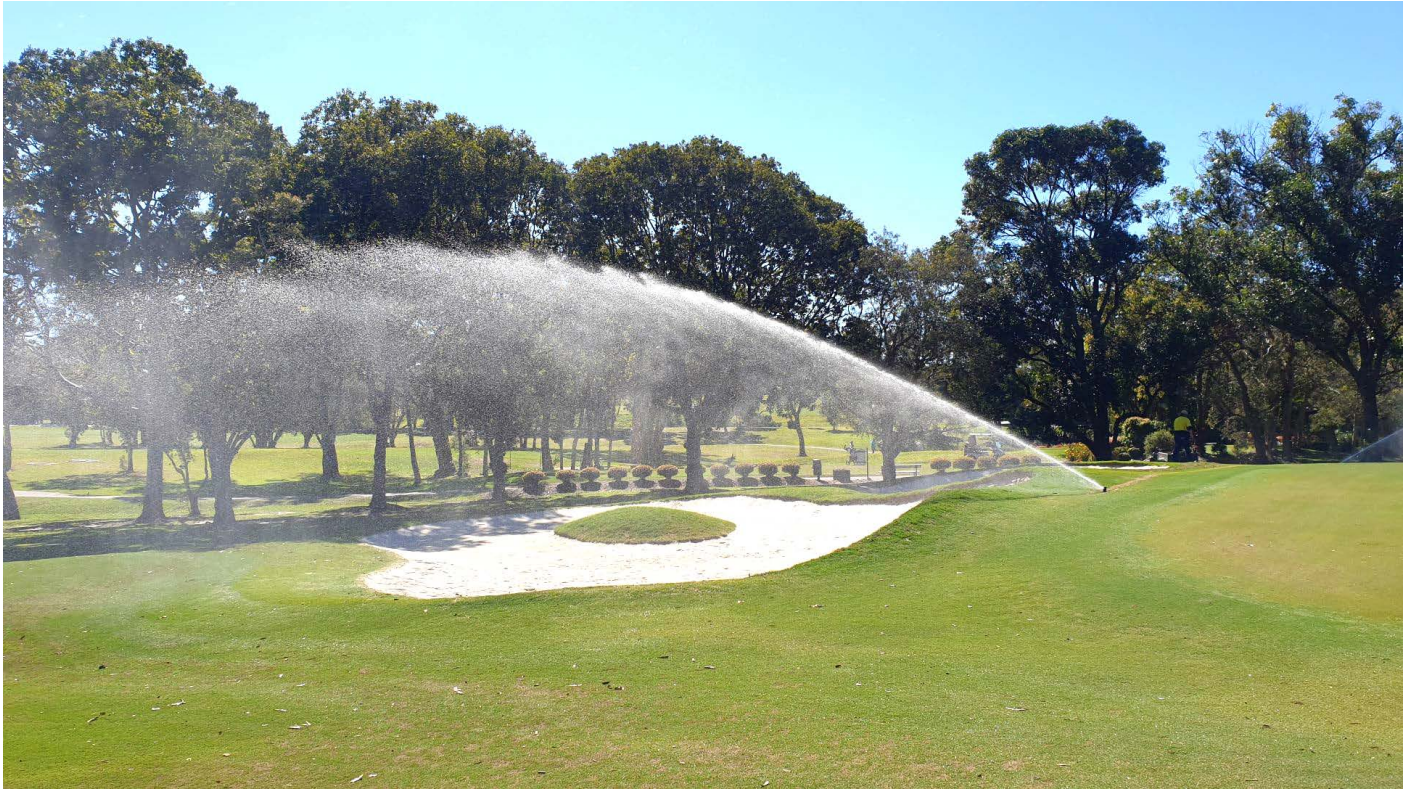
Hydro Vision's key sectors are commercial landscape, sports turf, public open spaces, pumping and filtration, stormwater harvesting and storage tanks, and golf courses. One of their recent projects was upgrading the irrigation system at Caloundra Gold Club, pictured here.
